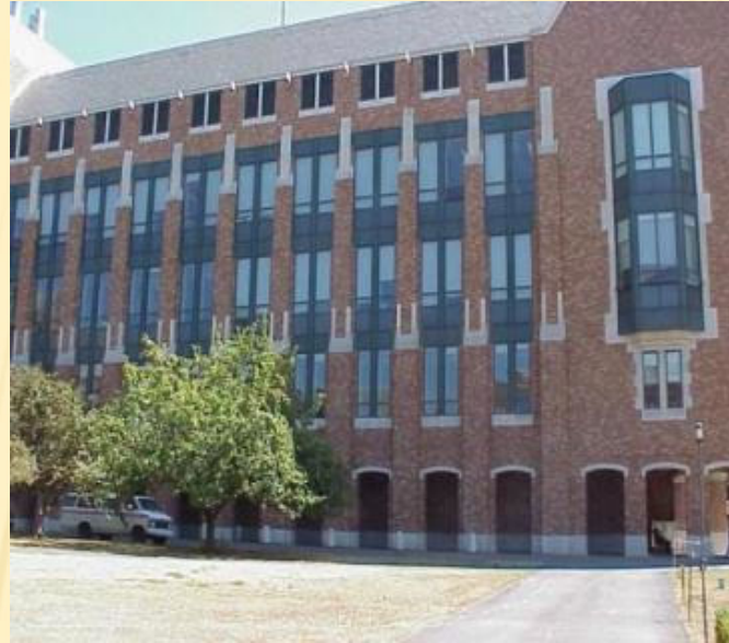
Upper story windows
