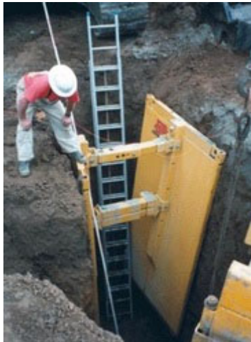
Figure A12.11: Trench box supporting excavation (Source: United Rentals, www.ur.com )
