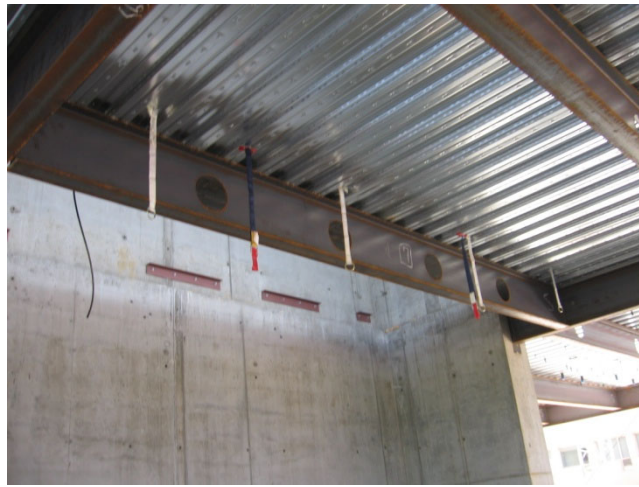
Figure A12.5: Concrete straps attached to slab reinforcement above
