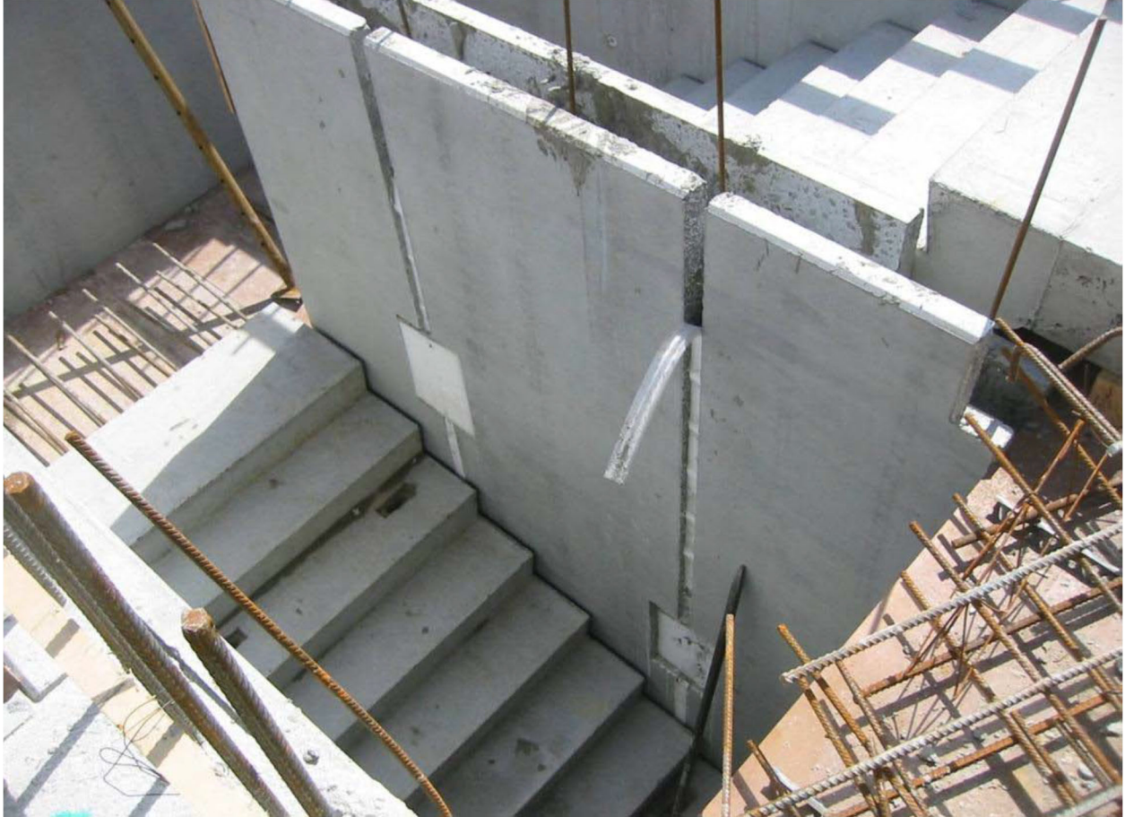
Figure A12.13: Precast spine walls and stairs under construction
