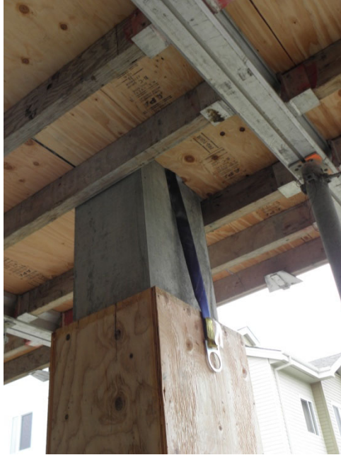
Figure A12.4: Concrete strap hanging below formwork from column reinforcement
