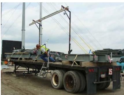
The photo to the left shows anchor posts with harness access being used by workers to unload steel from a flatbed trailer.
