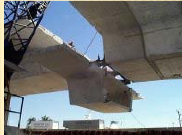
Concrete Segmented Bridge
