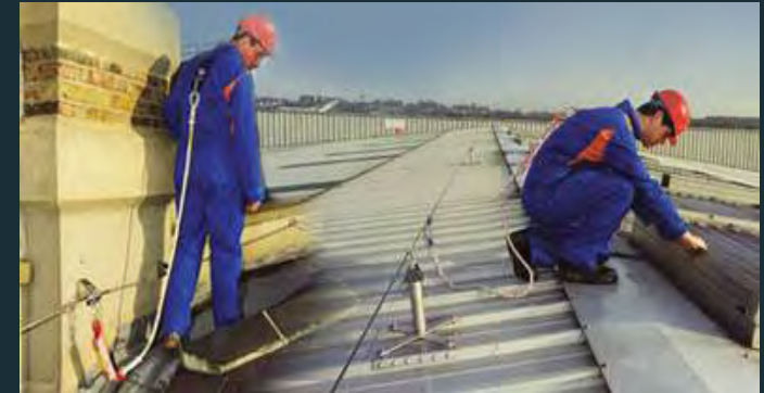
Mansafe cable and lanyard system
