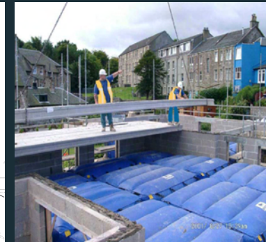
Sockets in slabs for edge panels
