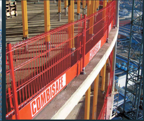
Sockets in slabs for edge panels
