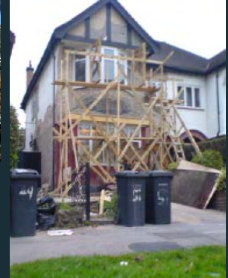
Proprietary scaffolding preferred
