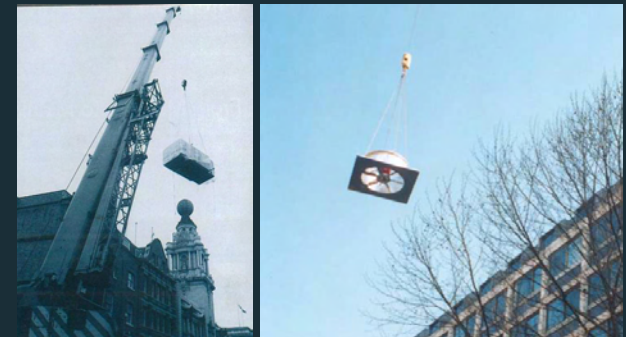
Vaults, trees and crane size issues
