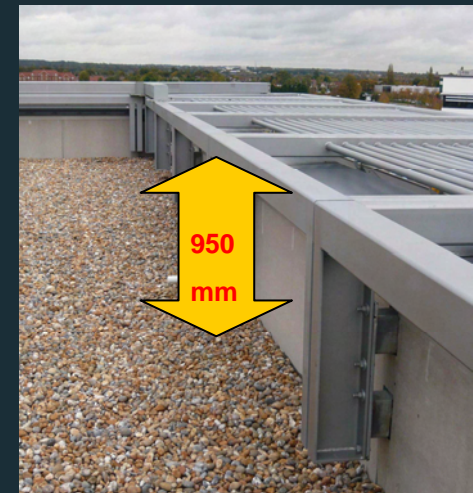
View of roof upstand
