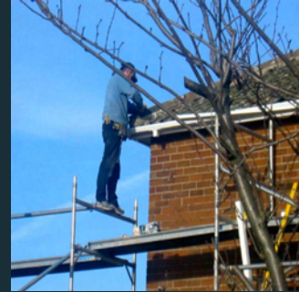
Scaffolding to be used appropriately
