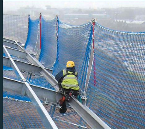
Holes in steel for net guards
