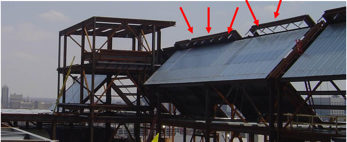
Figure7 - Roof davits installed early during the construction phase for contractor use throughout the project.
