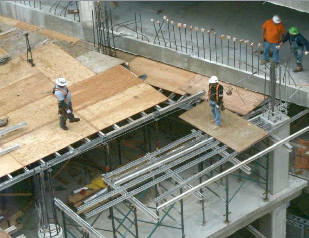
LEED Gold building under construction
