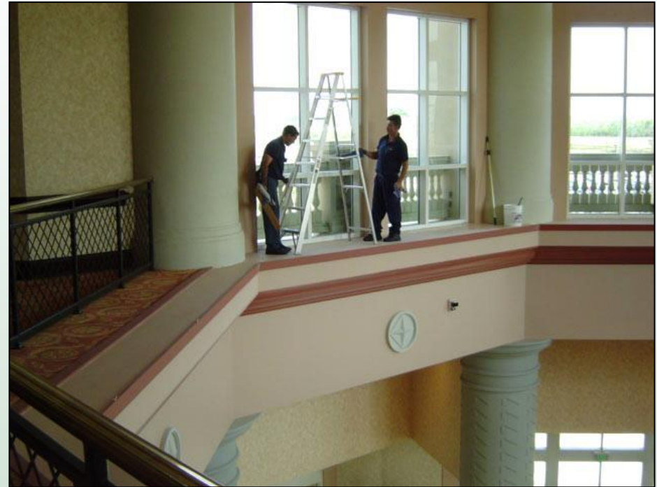
Fall exposures during Atrium Maintenance work. Photo: Mike Behm
