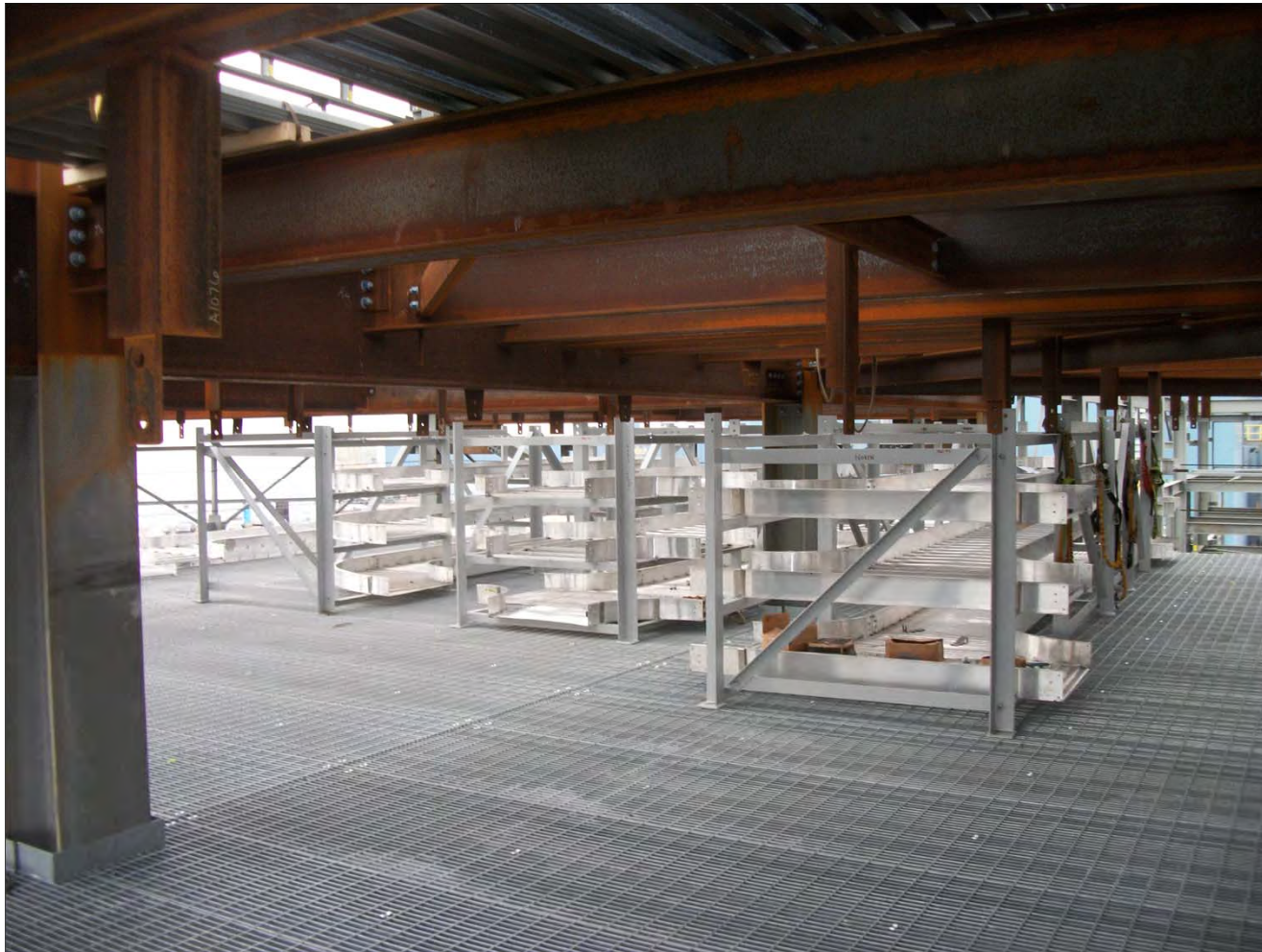
Tray bundles staged in cable tray spread area
